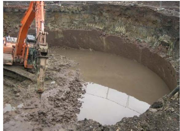
7. Excavation of the granular made ground to infilled gasholders. Infill was excavated to puddle clay layer (at circa 5.5m deep) and the clay excavated. Gasholder upfilled with granular materials loosely placed (as located beneath store footprint) for subsequent improvement by the installation of vibrated stone filled columns.
