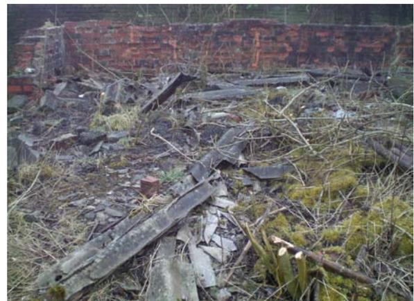
2. Vegetation and topsoil strip. This material was geotechnically unsuitable as a structural fill for reuse beneath proposed development areas and was removed from site.
